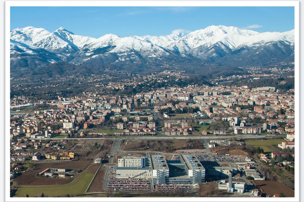
The New Biella General Hospital
